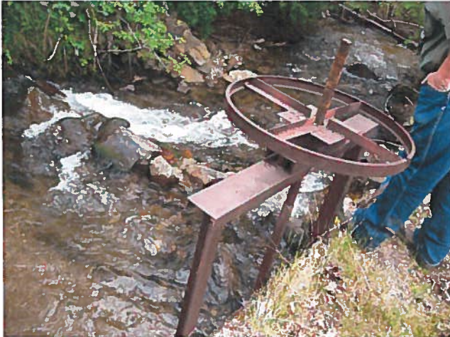
This is a photo of the ditch headgate.
