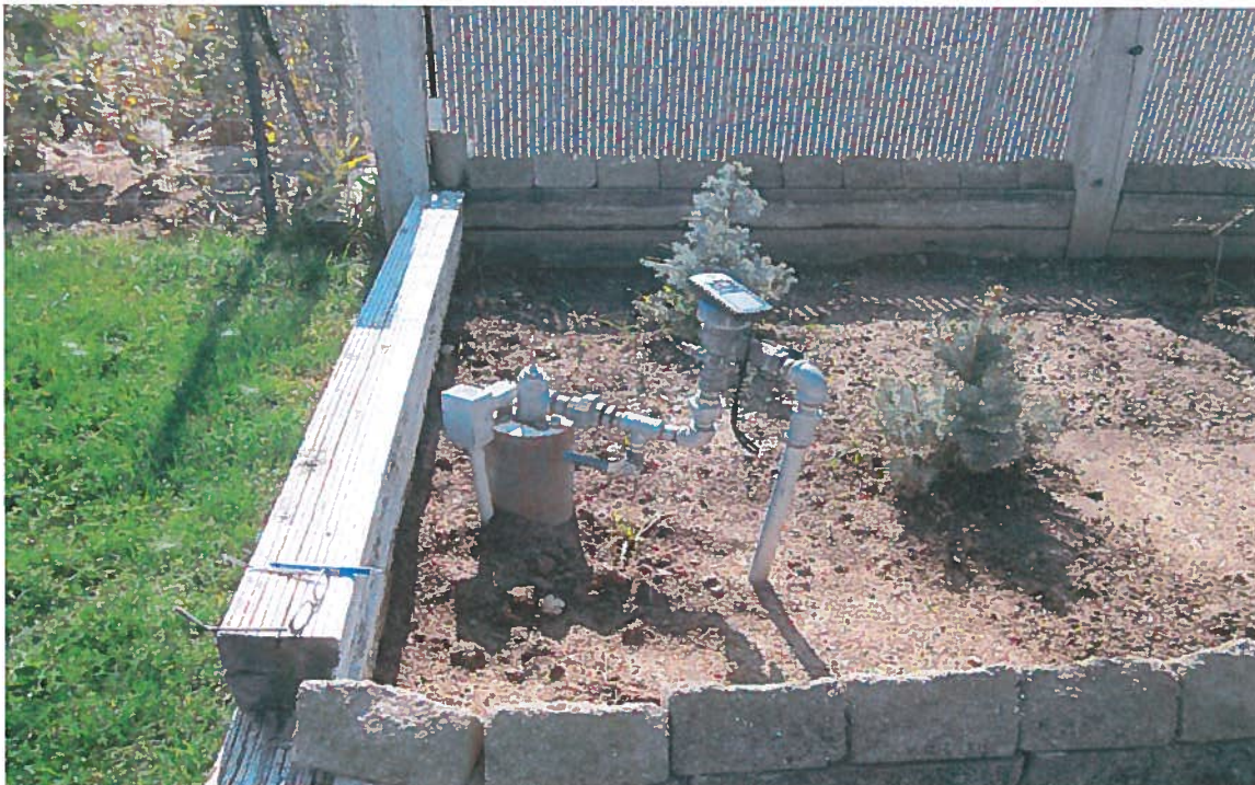
The water user refers to this as the “irrigation well”, however, it is a cased hole with a submersible pump. Water is pumped here from the domestic heating system, then used for irrigation in a sprinkler system.
