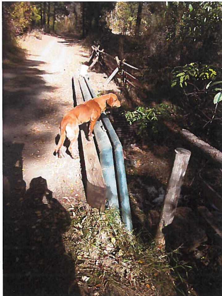
The smaller pipe shown in the photo supplies water to the pond. The larger pipe originates upstream in Indian Creek and provides water to the hydropower turbine downstream.
