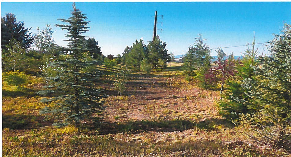
Place of Use: View southerly along State Highway 55 of landscaped area around Idaho Power substation.
