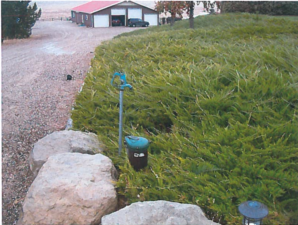
63-32827 Exam 10/22/2012: POD area. POD well buried within shrubbery approximately 15 ft from the new well (serves in-house domestic and lawn irrigation uses) in photo foreground facing north. Barn in photo background where “pump room” located.
