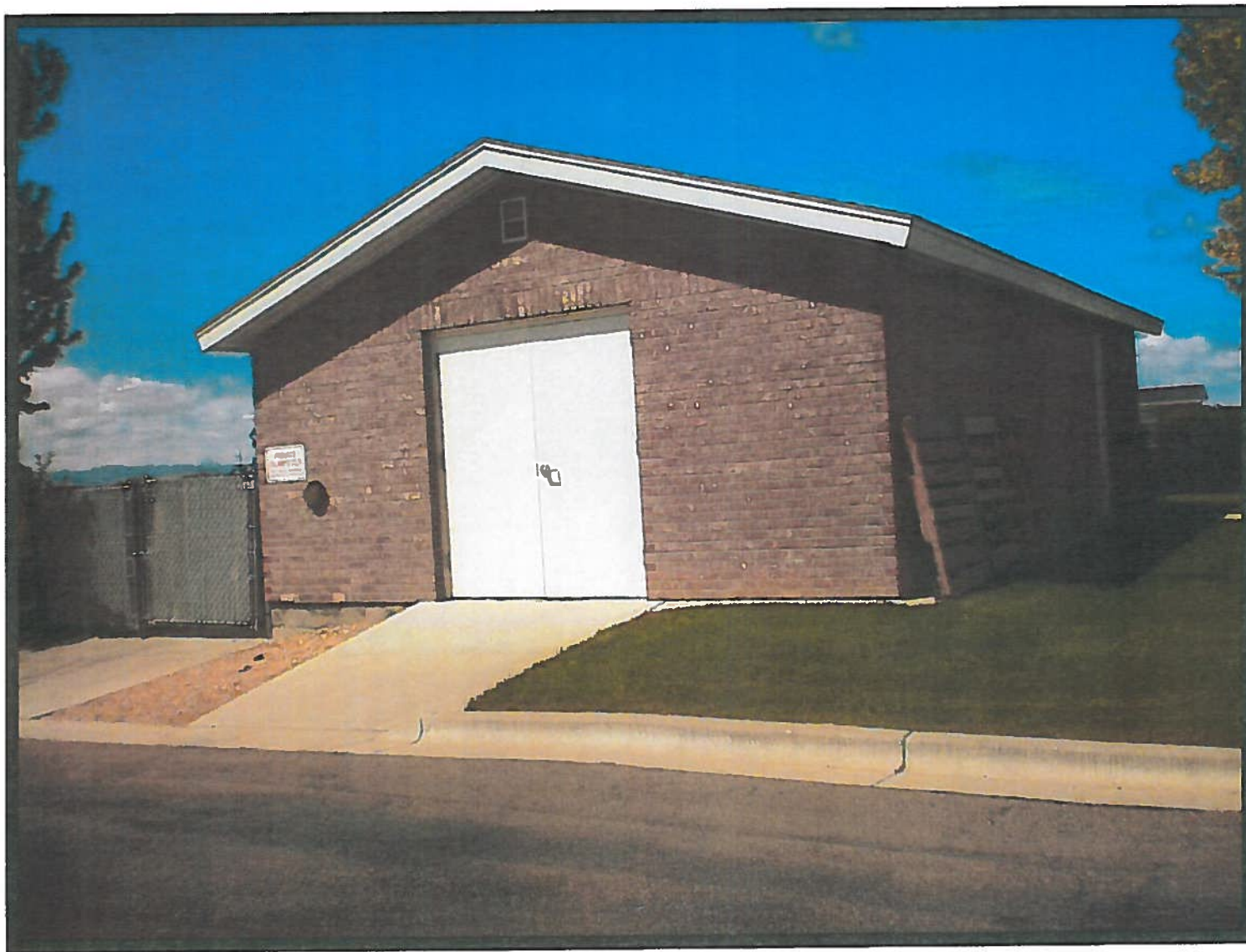
Well and pump house
