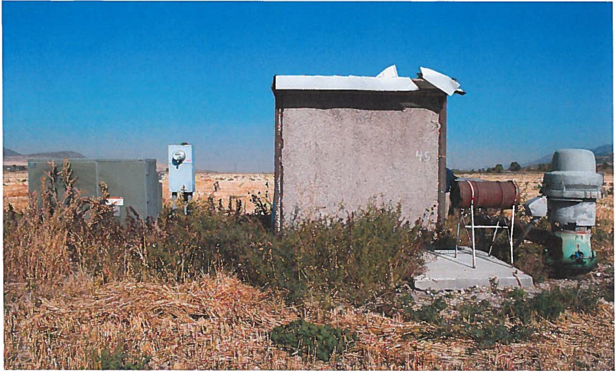
Back Side of well and Pump house
