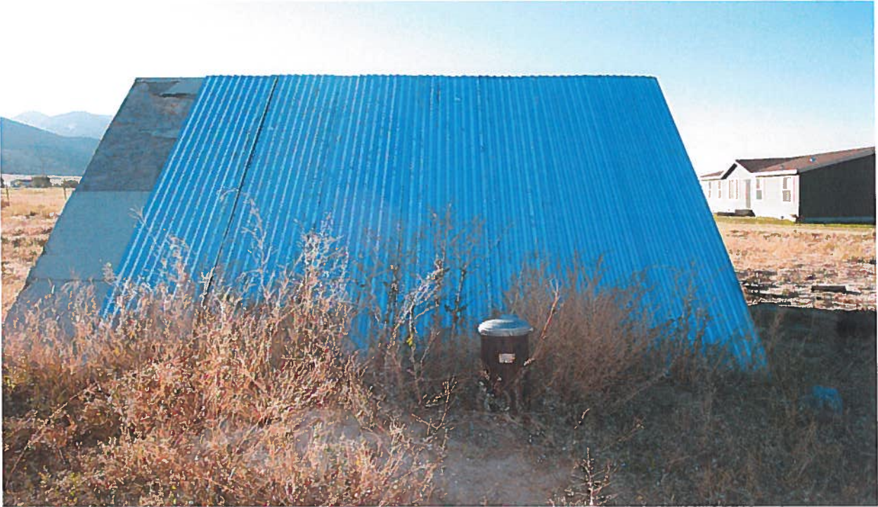
Well & Pump house
