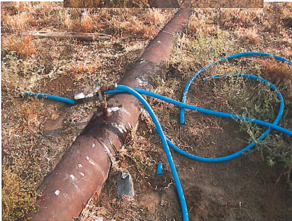
This is a photo of the 1st split off the mainline. I attempted to take a pressure reading here but my gauge maxed out at 100psi and the pressure was greater than that.
