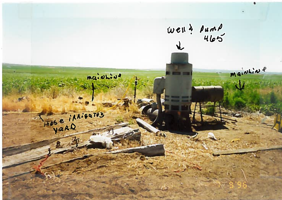
Well # 465. Pump Diverts water into a North & South mainline that feeds the handlines
