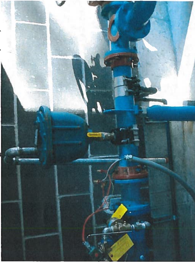
Photo #10. Pressure reducing & Solenoid shut-off valve (Blue)
