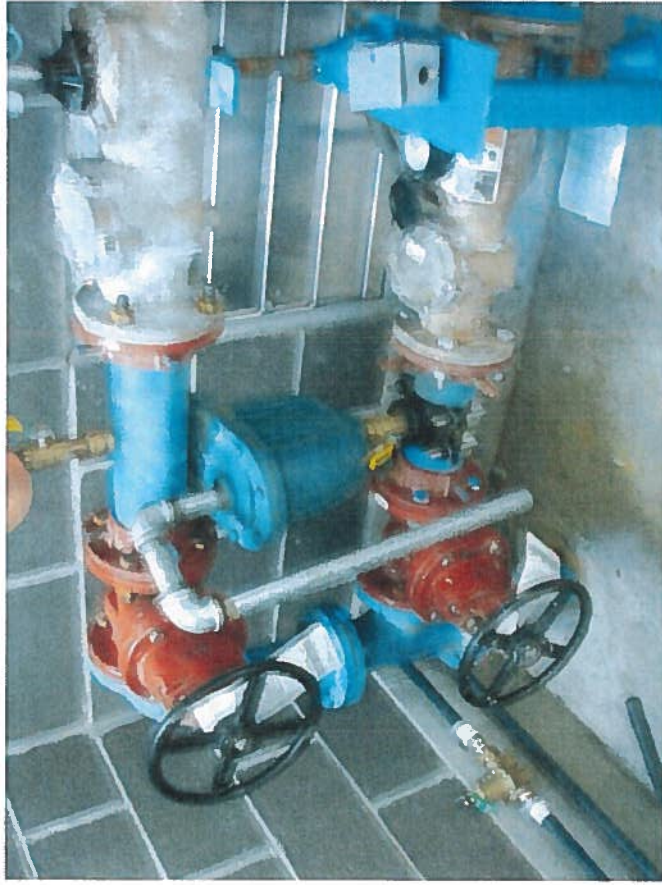
Photo #9. New pump house/chlorinator building piping & vent
