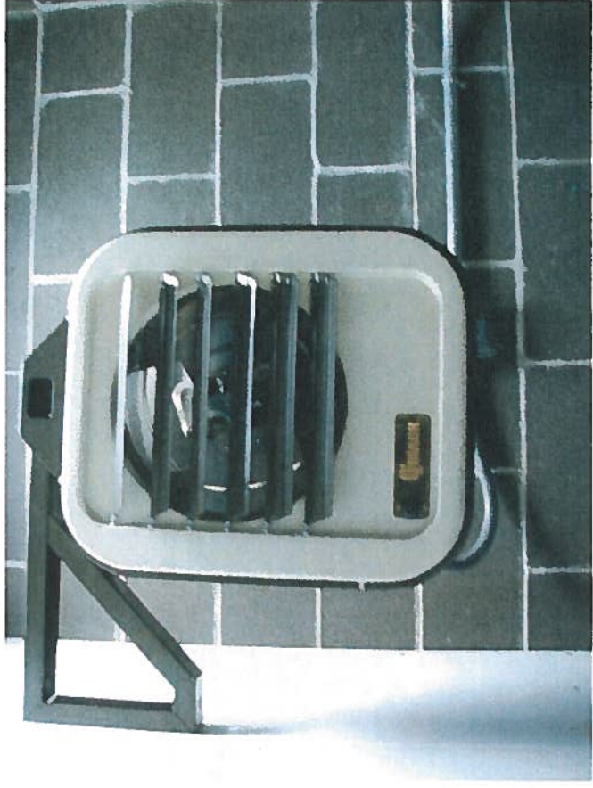
Photo #14. Chlorine building heater
