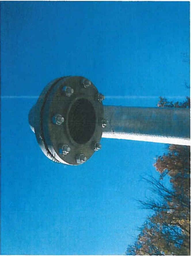
Photo #5. Tank #2 30,000 gallon, new hatch and vent
