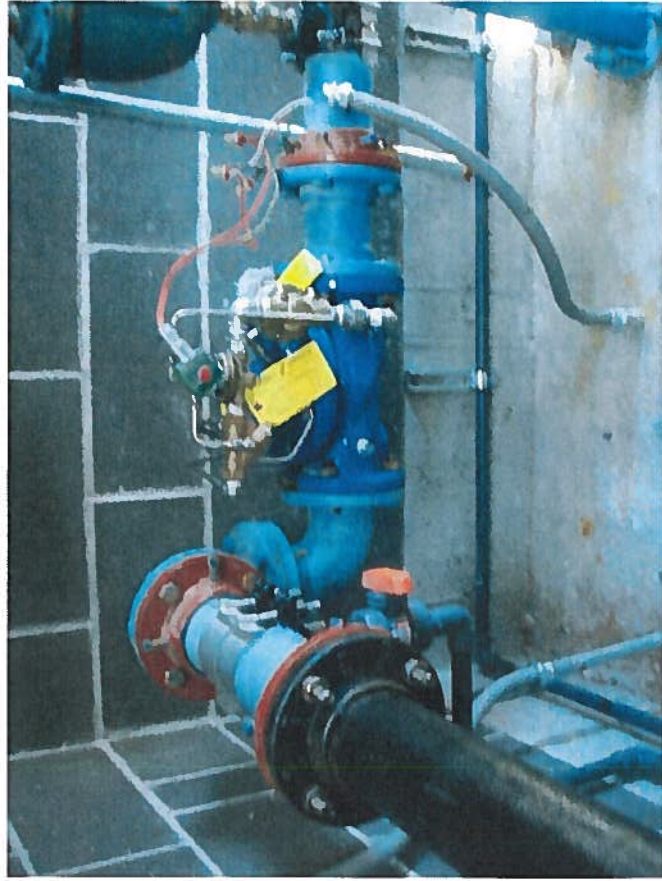
Photo #10. Pressure reducing & Solenoid shut-off valve (Blue)
