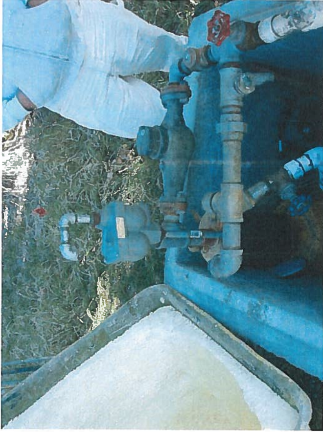
#42. Well 3 piping, vent, flow meter, sample tap, & isolation valve
