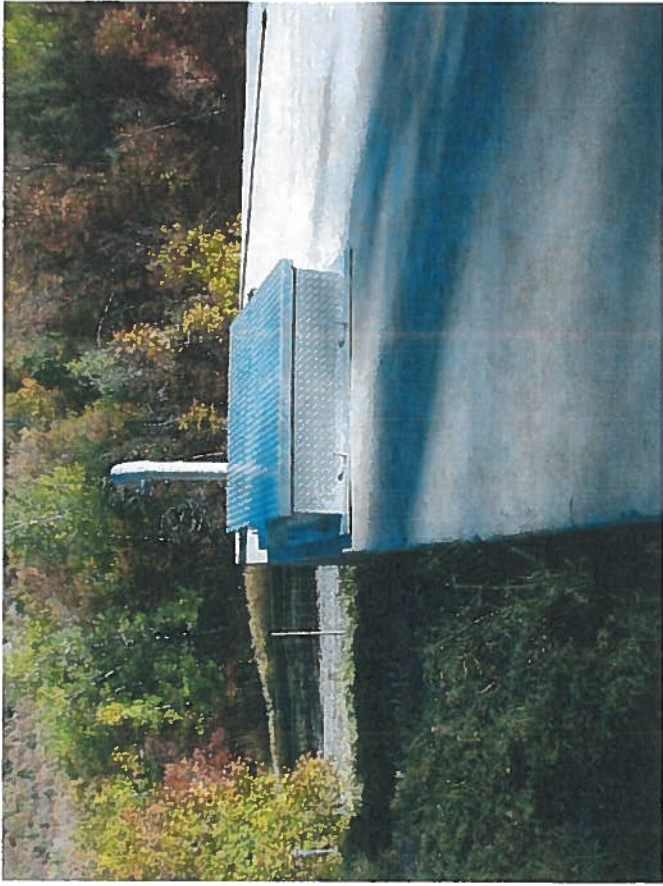
Photo #5. Tank #2 30,000 gallon, new hatch and vent
