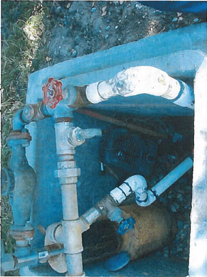
#42. Well 3 piping, vent, flow meter, sample tap, & isolation valve
