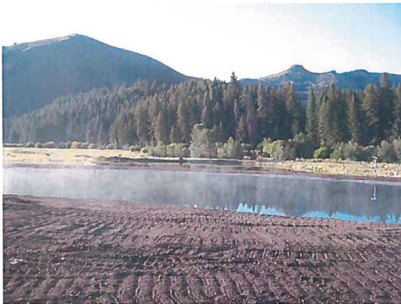
Small pond just after construction, looking south-southeast – 8/5/11
