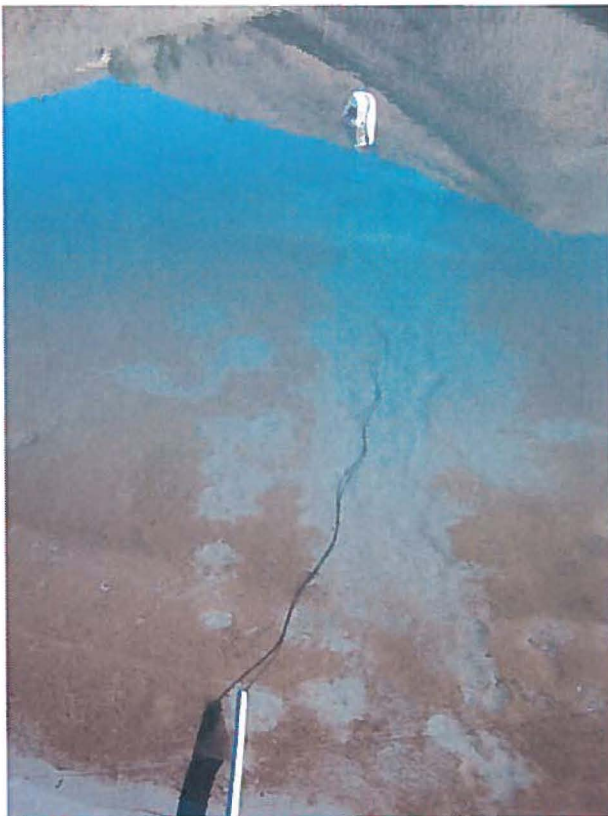
Temperature sensor and float – 10/29/2012
