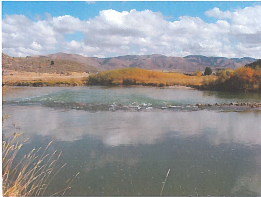
Figure 1 Rock barrier in Bear River
