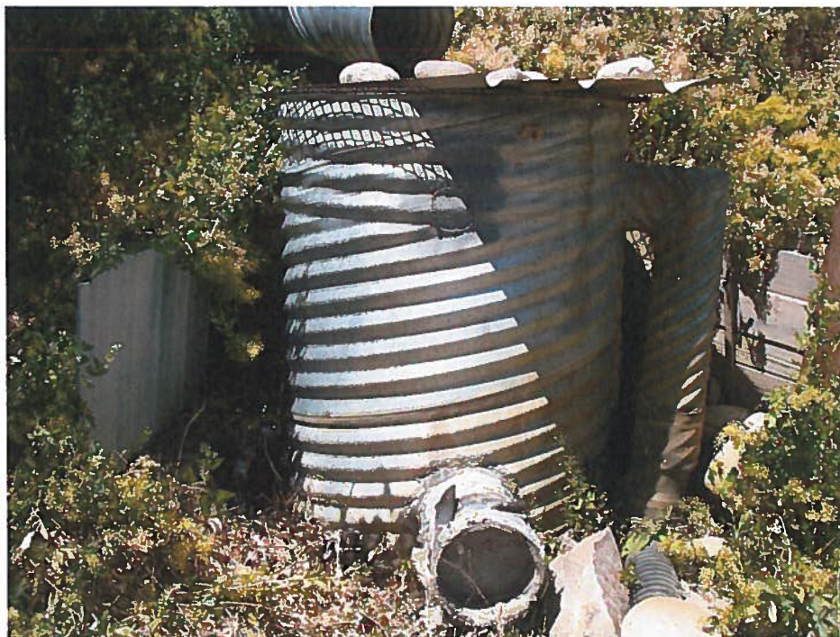
65-22940 Exam 7/18/2012: 12 in corrugated pipe from spring, under road, into 400 gallon tank. One of 1 in discharge lines visible coming out bottom left of tank.
