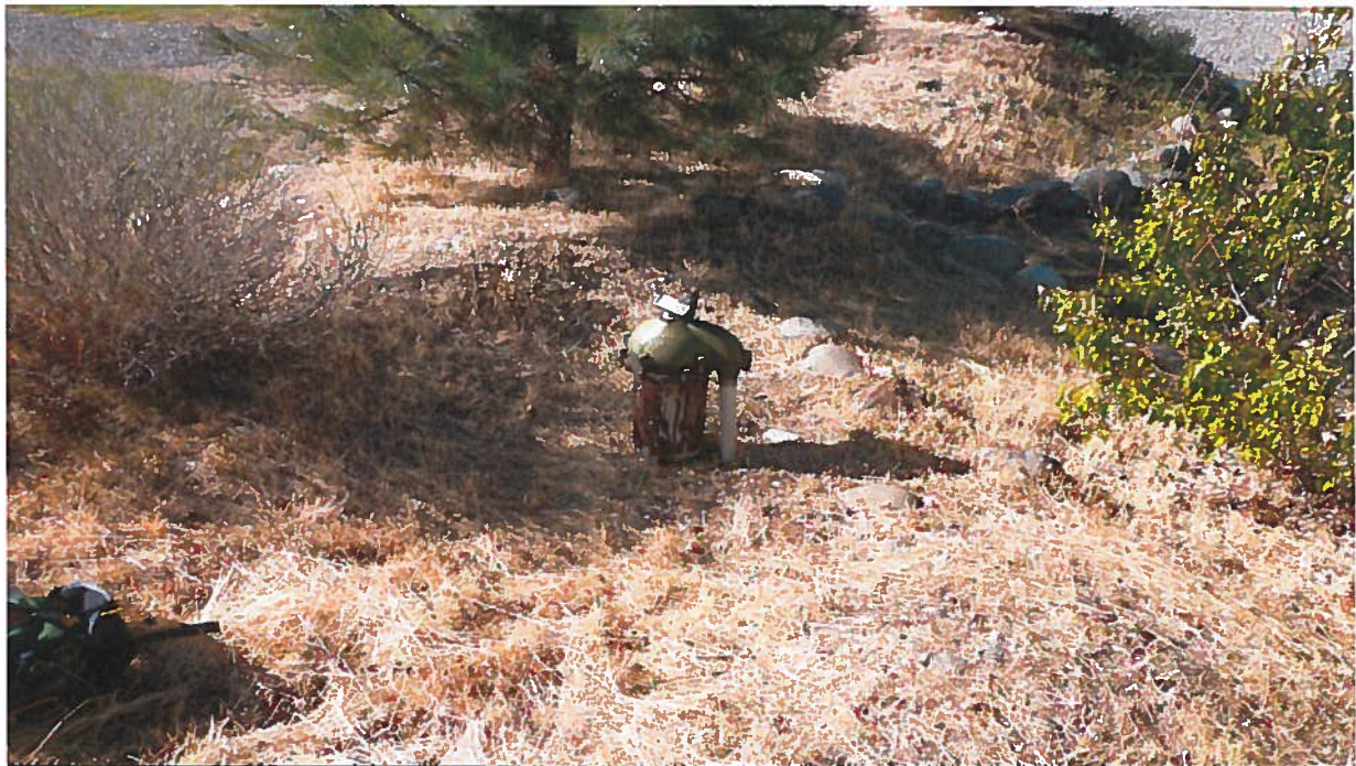
Point of Diversion: View southwesterly of domestic ground water well. Well is used for supplemental irrigation of RV sites when main diversion in Little Salmon River cannot meet the irrigation needs of the RV park.
