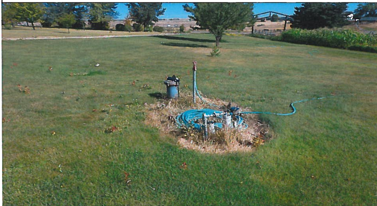
Point of Diversion: View northerly of ground water well and irrigation control valves.
