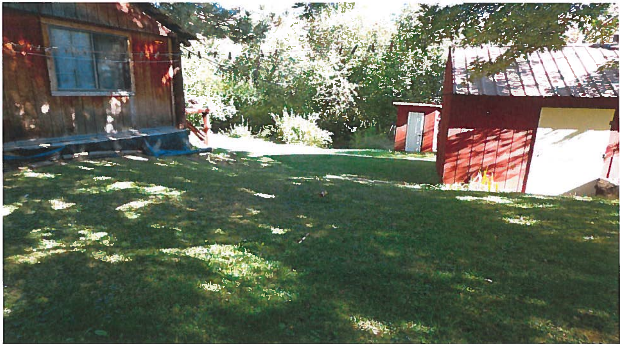
Place of Use: View northerly of lawn area and sprinkler irrigation. Sprinkler hoses are attached to risers spaced along the 6" PVC conveyance pipe.
