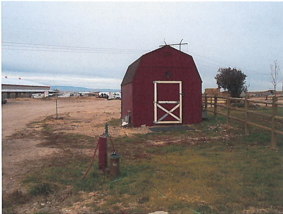
63-32899 Exam 10/26/2012: POD well with pump house/shed in photo middleground facing west. Portion of large barn (commercial POU) left side of photo.
