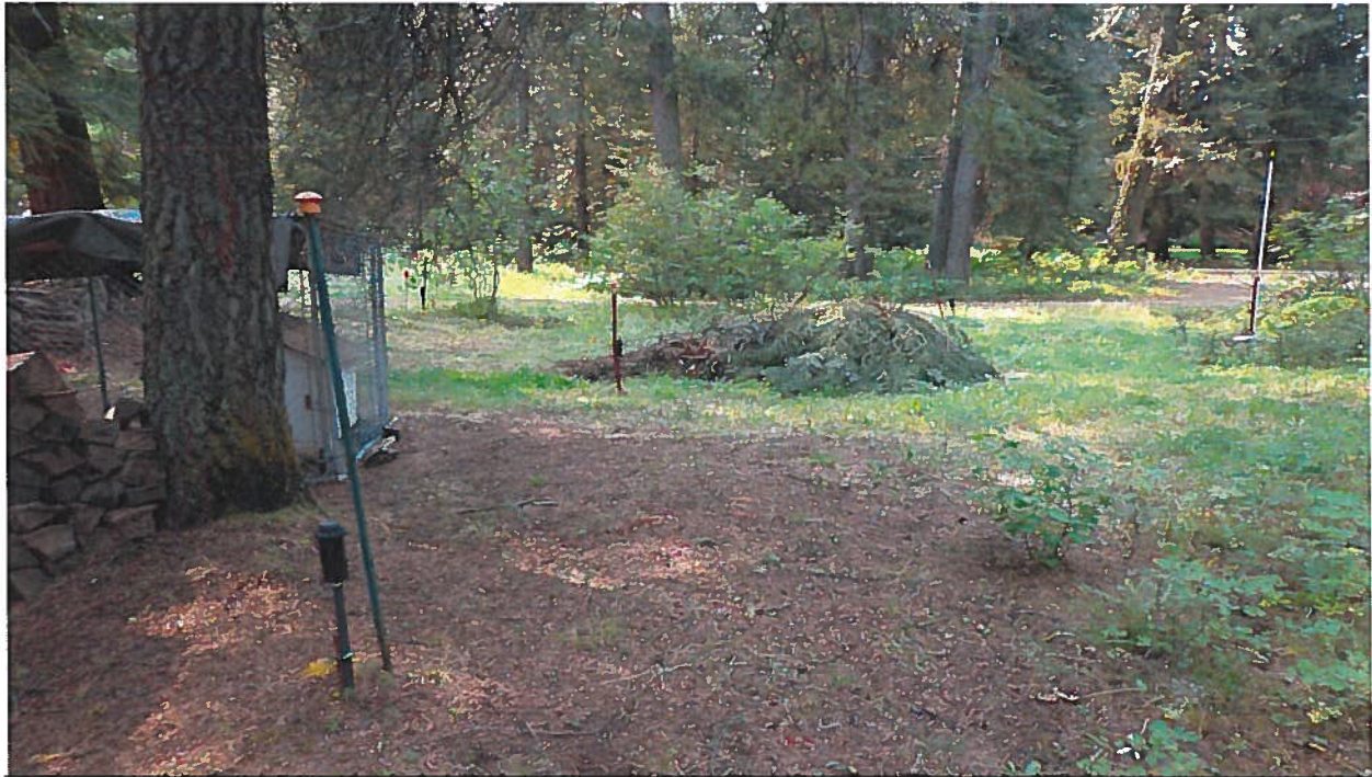
Place of Use: View southerly of typical sprinkler risers located within the property to irrigate the native vegetation areas.
