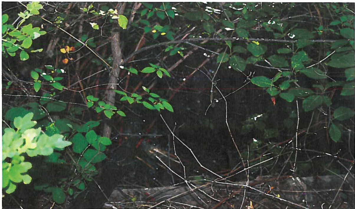
Pipe back into creek, just above the recreation storage pond
