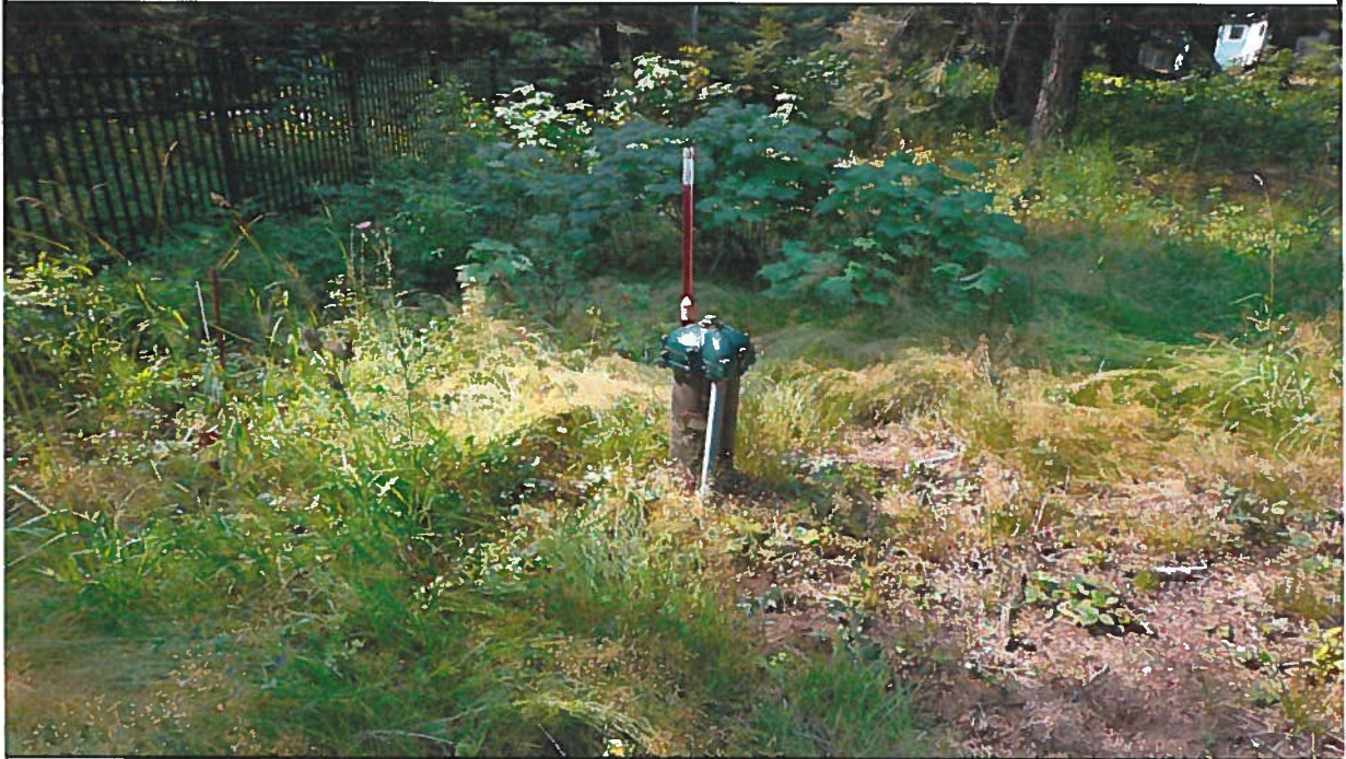
Point of Diversion: View southwesterly of ground water well located near the easterly lot line.
