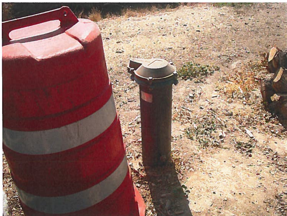
63-33272 Exam 8/27/2012: Injection well facing south. Injection well usually covered by/underneath the adjacent orange construction barrel.
