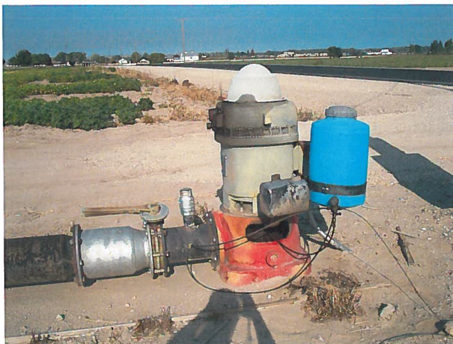
63-11851 Exam 8/30/2012: POD facing west.
