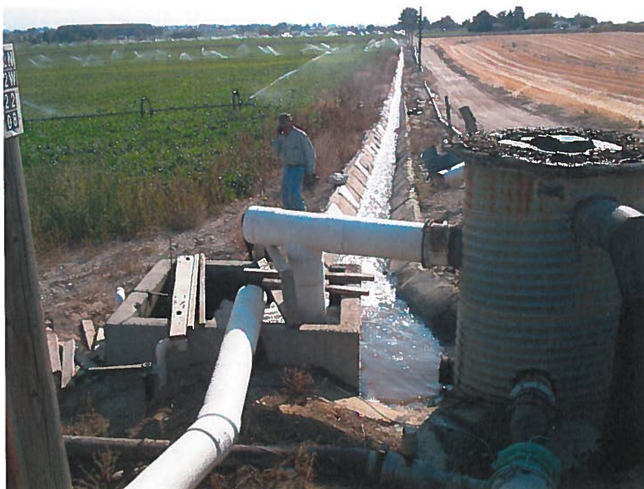
63-11851 Exam 8/30/2012: Location where water discharges from well into cement ditch at top of hill (southern most edge of POU). Portion of booster pump visible in right side of photo foreground. Cement box visible where water diverted for surface water irrigation. Portion of POU left side of photo, sprinkler irrigation with surface water occurring during exam. All water in cement ditch at time of exam from well.
