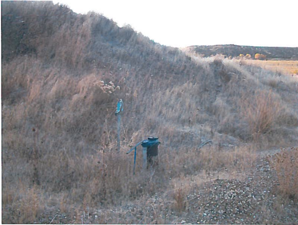
63-31631 Exam 10/26/2012: POD well facing south/southeast.
