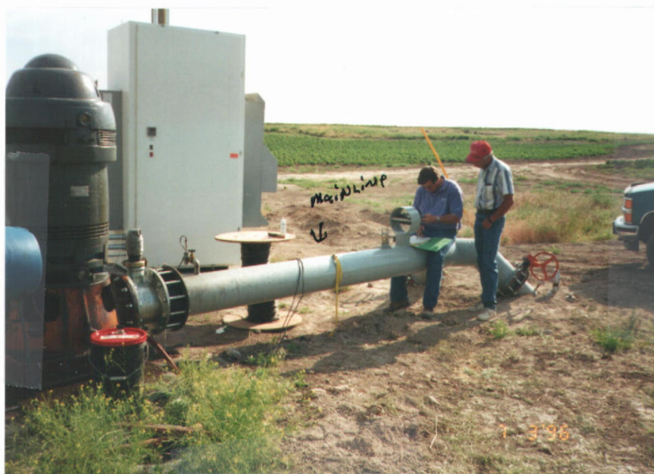
This is The Diversion works FOR well, IT SPLITS INTO TO main lines at The POINT Where The man is sitting on The pipe. OCT 03 1996
