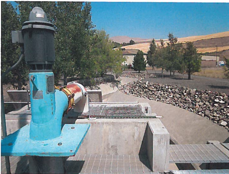
Photo #6. S-Curve raceways.
