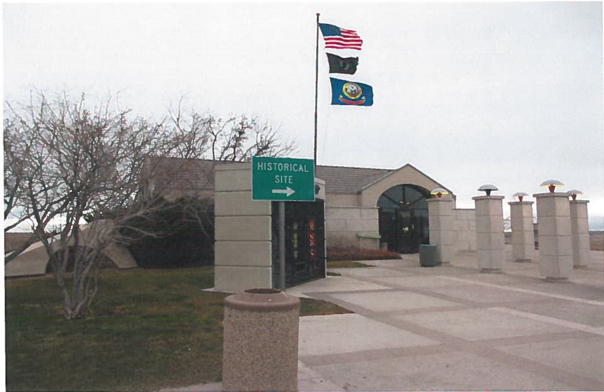
Rest Area Building and Lawn
