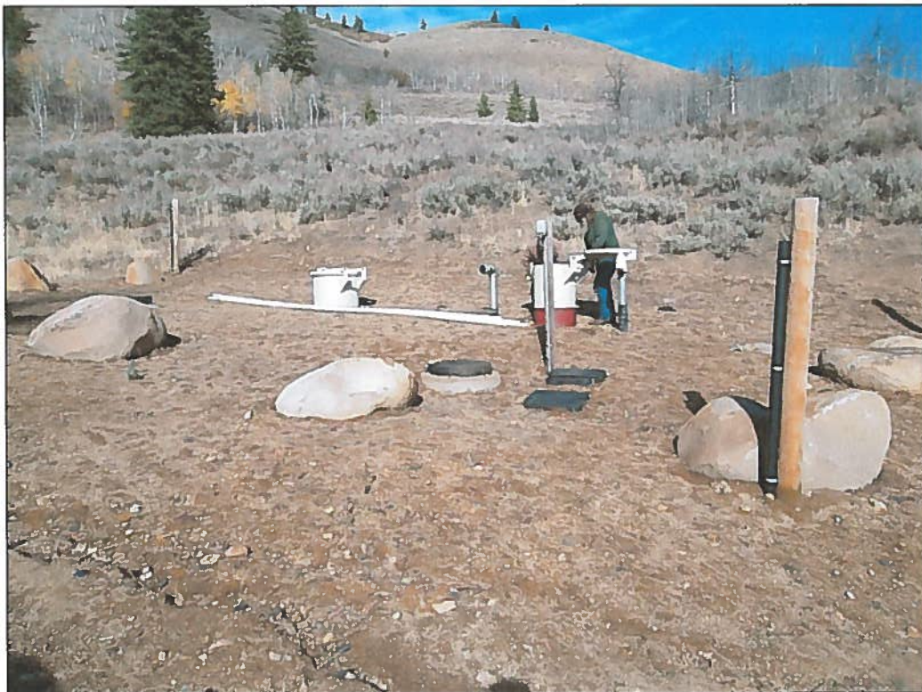
Buried 10,000 gallon tank, looking north
