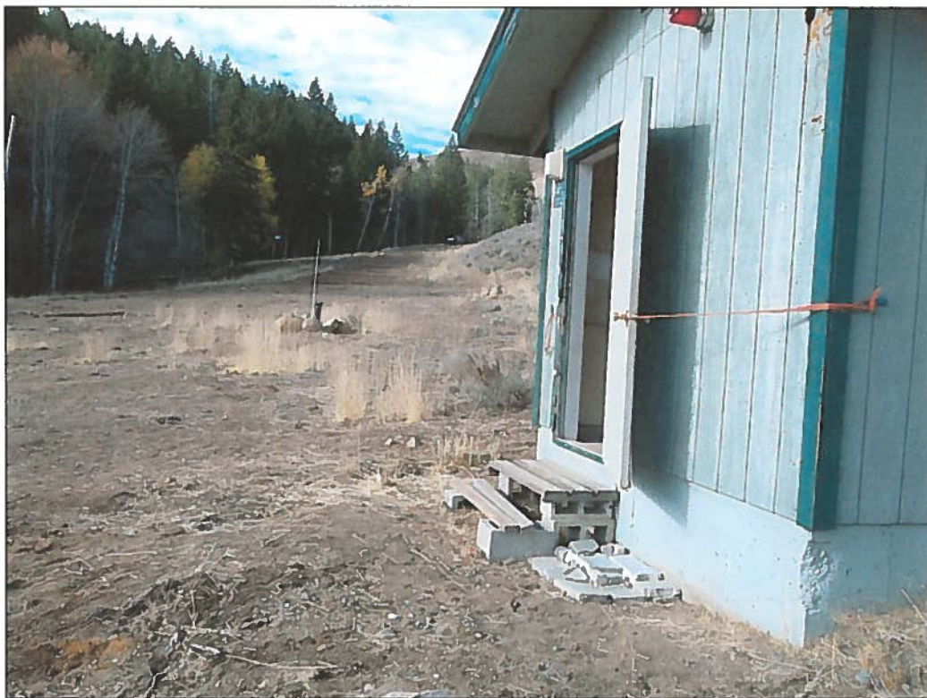
Wellhouse in relation to wellhead, looking west
