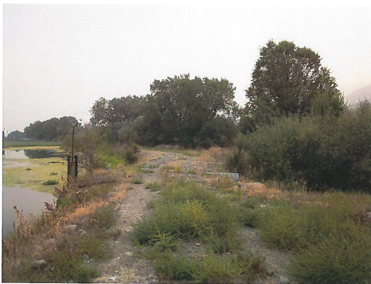
Headgate for water leaving the pond
