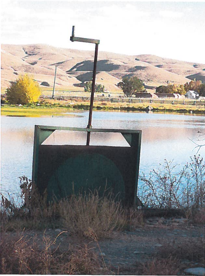
Headgate looking east, southeast
