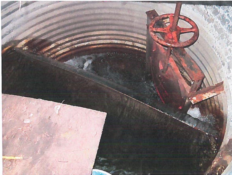
Figure 2: 6' sharp crested weir below ponds
