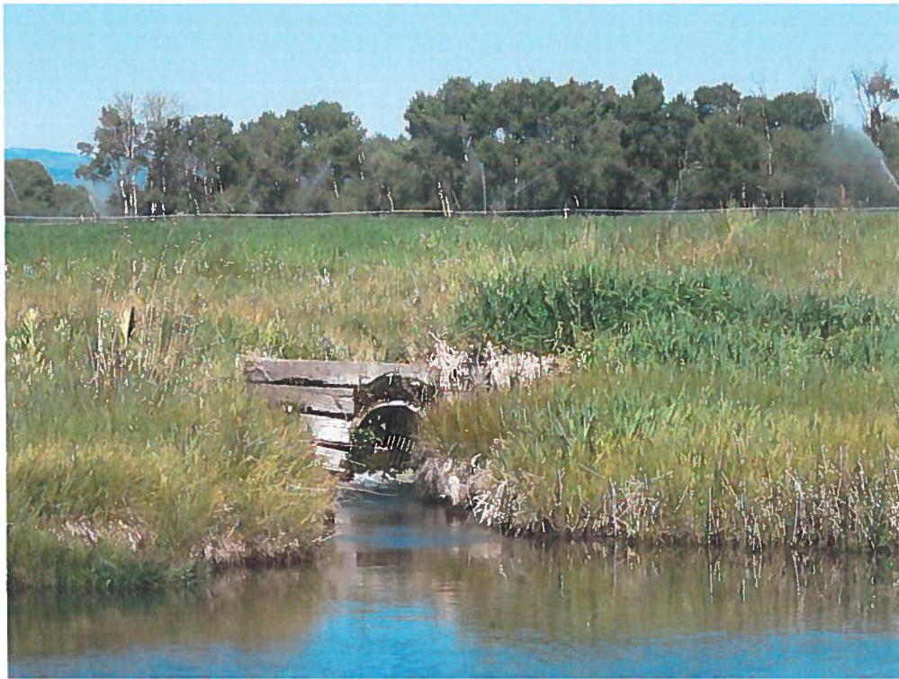
Figure 5: Point of injection on Loving Creek
