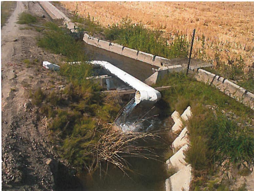
63-33147 Exam 8/30/2012: Location where water discharges from 8" gated pipe into small pool area from which water crosses over weir into cement ditch.
