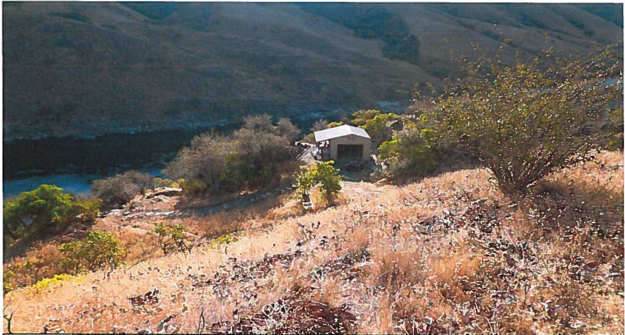
View southeasterly from the location of the 4,000 gallon and 1,200 gallon water storage tanks of a storage building which houses the pump controls.
