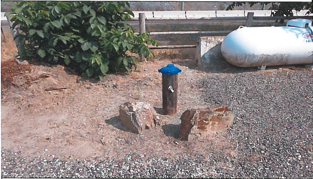
Point of Diversion: View easterly of ground water well. A pump house is located approximately 15-feet south of the well.
