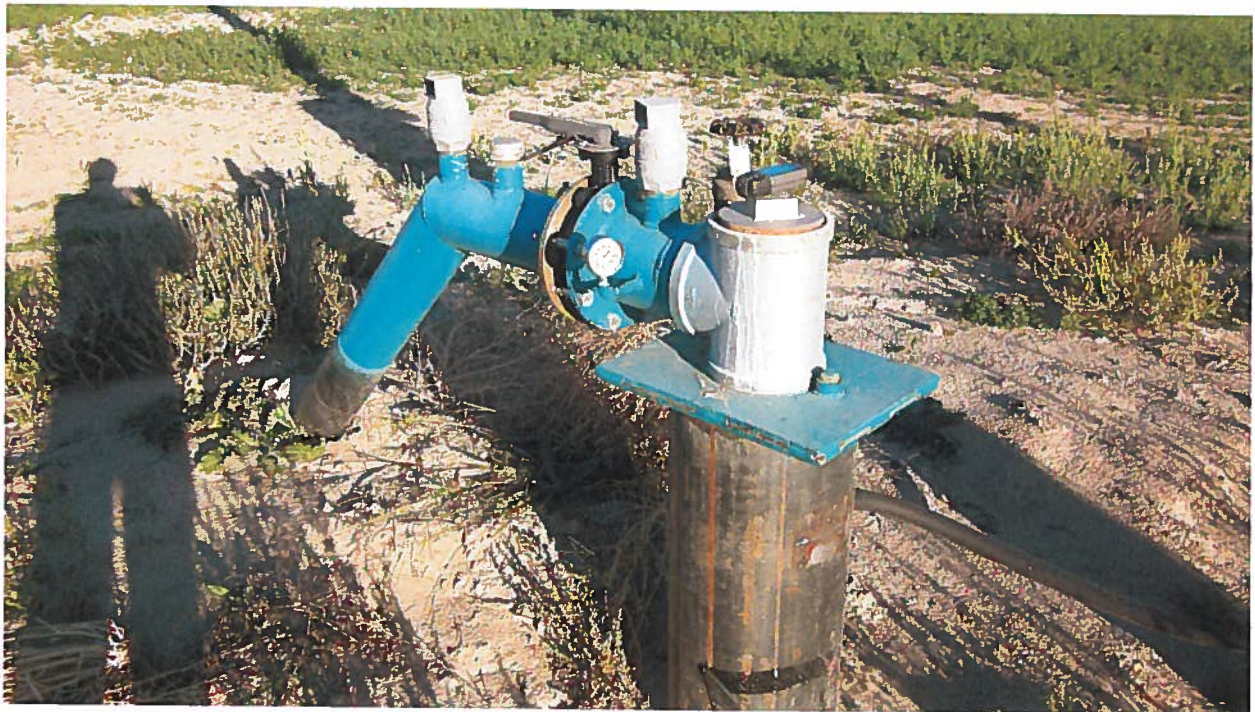
Photo 2. View of POD with pressure gauge.
