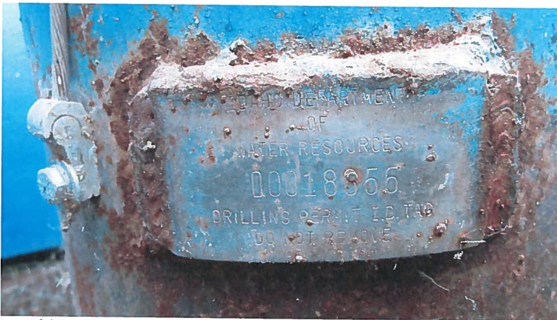
Close-up of the well ID tag, D0018856.
