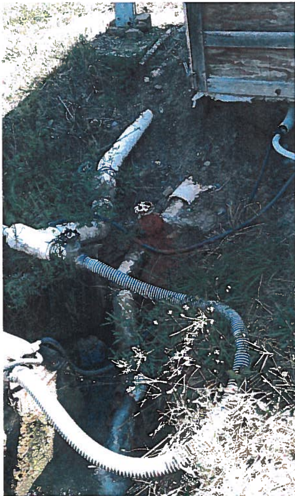
Discharge back into the river
