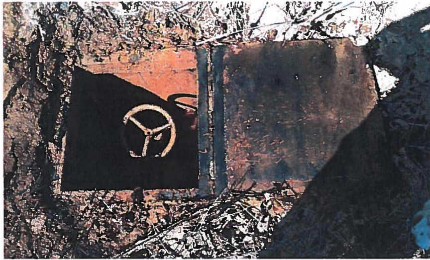
Diversion valve with box.
