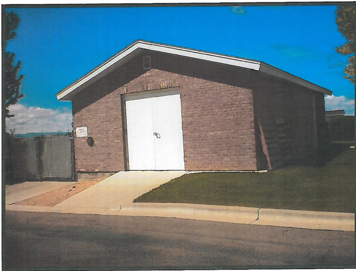
Well and pump house
