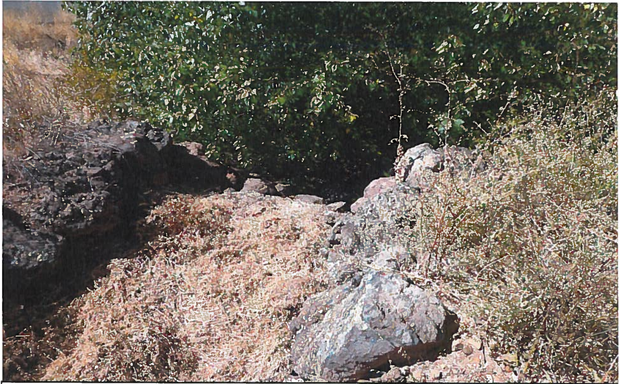
View westerly of aesthetic pond spillway channel on Cool Creek.
