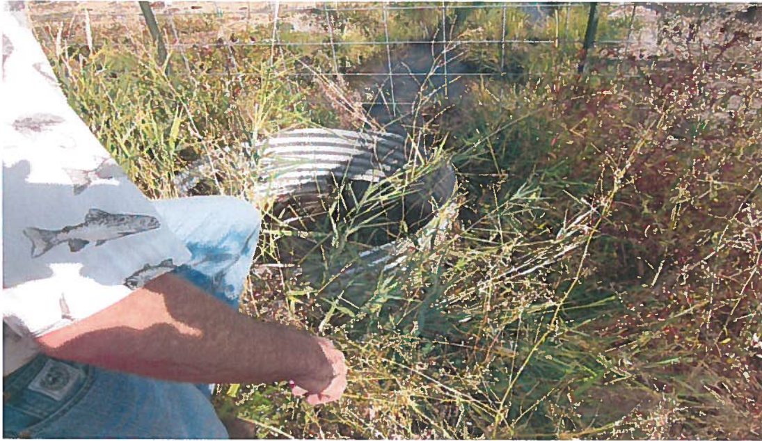
Corrugated pipe located in the northeast corner of the 4 lots.
