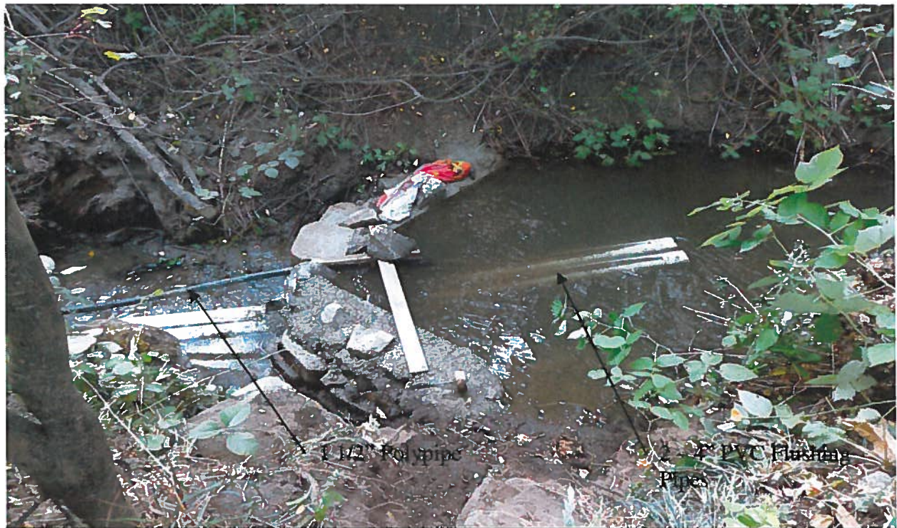
Point of Diversion: View southerly of 2 foot high dam constructed of concrete, rocks, and landscape blocks. The two 4 inch diameter PVC pipe sections are used to convey/flush water downstream of dam and to prevent overtopping of dam. The black pipe is 1 1/2" polypipe used to convey water to the 1,400 gallon irrigation water storage tank.
