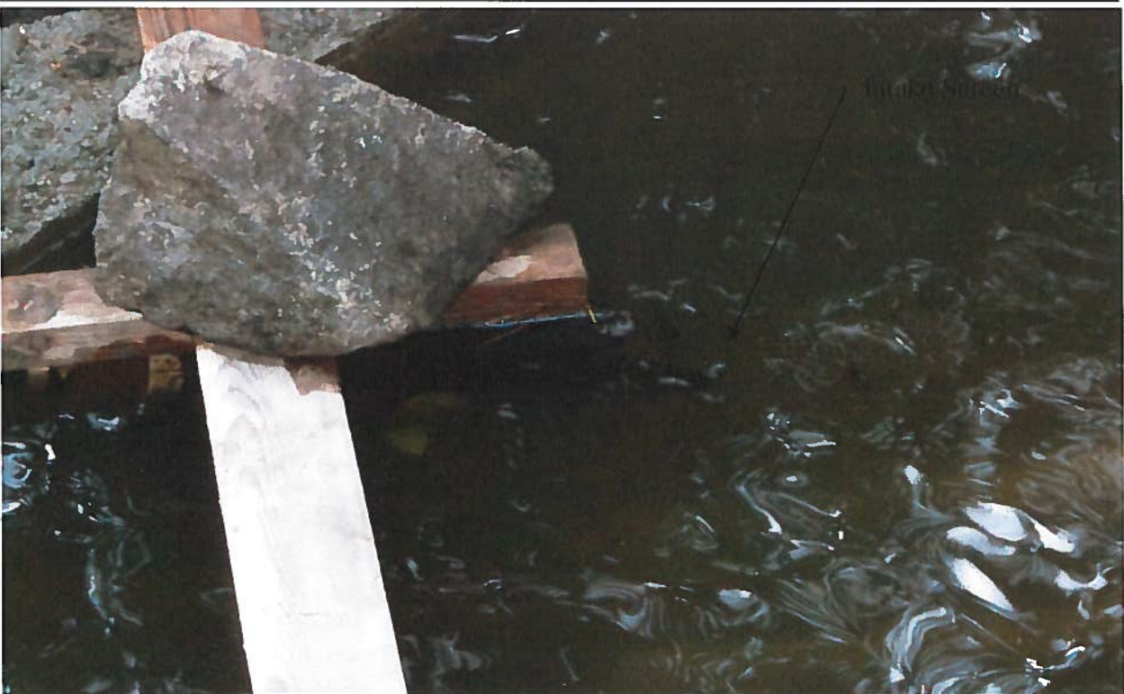
Point of Diversion: View of the intake screening for the 1 1/2" polypipe.
