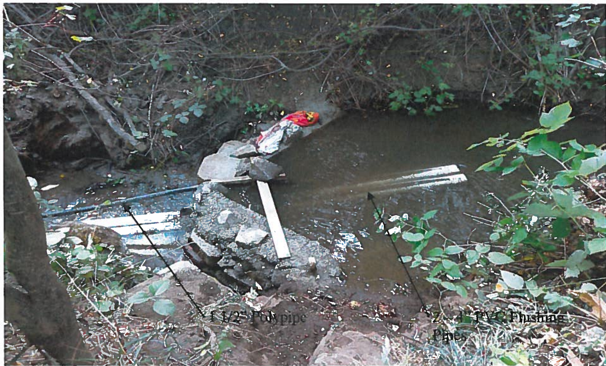
Point of Diversion: View southerly of 2 foot high dam constructed of concrete, rocks, and landscape blocks. The two 4 inch diameter PVC pipe sections are used to convey/flush water downstream of dam and to prevent overtopping of dam. The black pipe is 1 1/2" polypipe used to convey water to the 1,400 gallon irrigation water storage tank.
