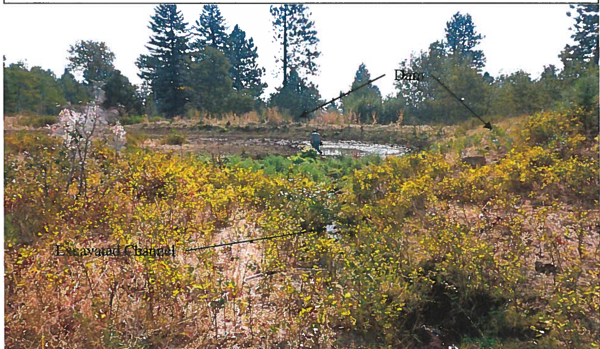
Place of Use: View southeasterly of stock water and fire protection storage pond. The dam height is approximately 7'. The excavated water conveyance channel from the 10" headgate on the roadway culvert is shown in foreground.
