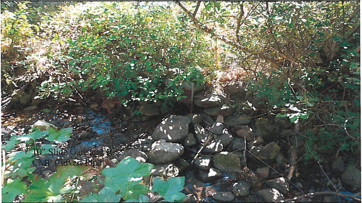
Point of Diversion: View southeasterly of 10" slide gate on 10" CMP culvert. The unnamed stream is known locally as Wilson Creek.
