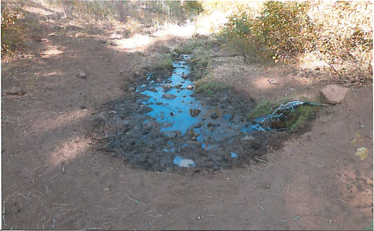
View easterly of the 1 ¼" galvanized steel water trough overflow pipe. The overflow is conveyed in a natural swale and percolates downstream into the soil.
