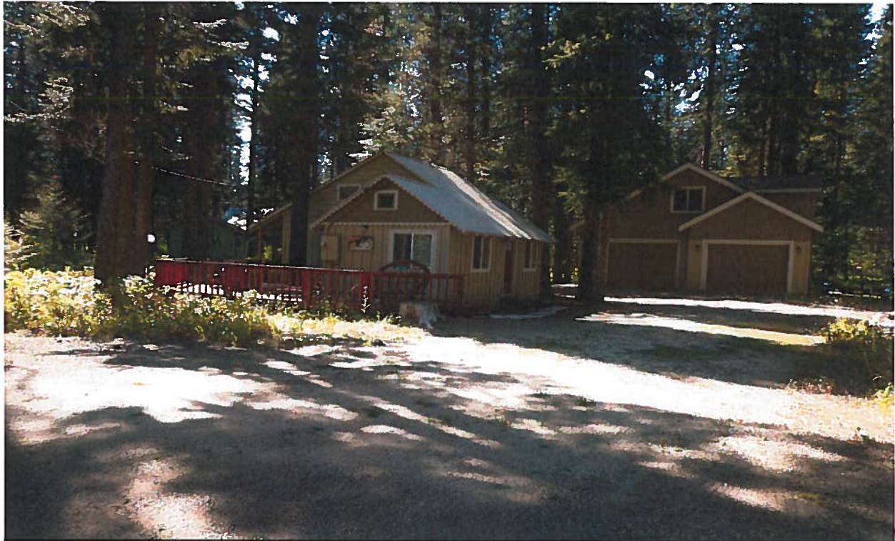
Place of Use: View westerly of cabin and garage located on Lot 10, Block 4, Pilgrim Cove Subdivision.
