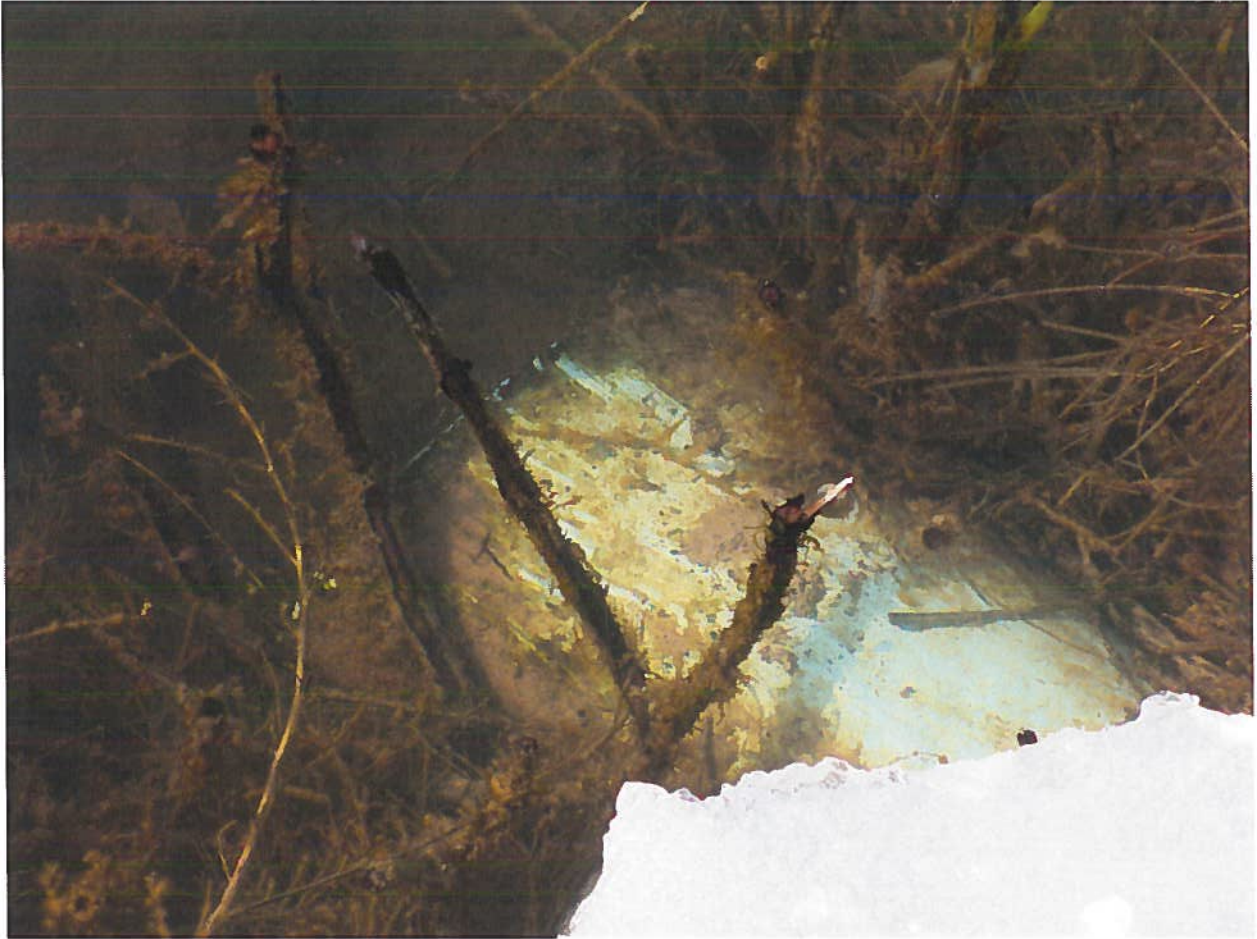
Submerged PVC Delivery Pipe in Pond
