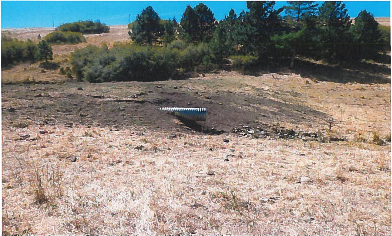
Place of Use: View southwesterly of the dam and the 24" diameter CMP culvert overflow pipe.
