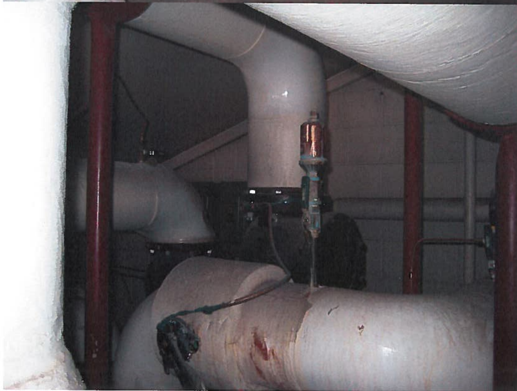
Part of diverting works
