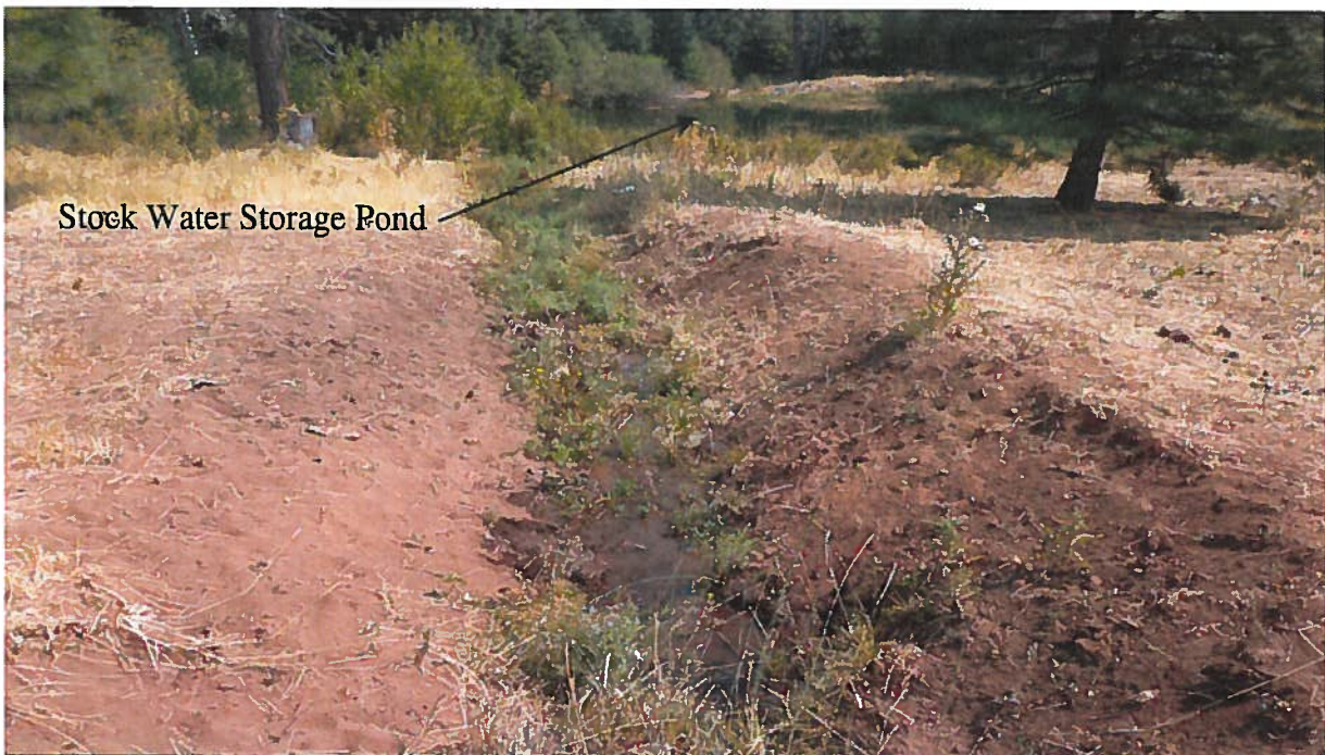
View northeasterly from point of discharge for the 1" PVC pipe into an excavated channel discharging to a stock water storage pond.
