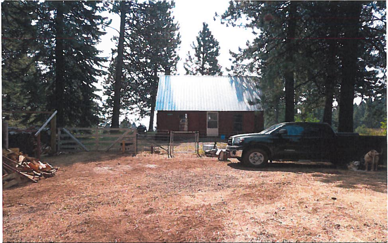
Place of Use: View southeasterly of the right holder's cabin. Spring water is diverted to the cabin by approximately 500 lineal feet of 1 ½" PVC pipe from the spring box.
