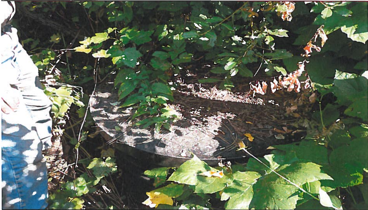
Point of Diversion: View of spring box. Spring box is constructed of 4' diameter plastic pipe with steel lid. The spring serves two homes for domestic use and lawn irrigation.
