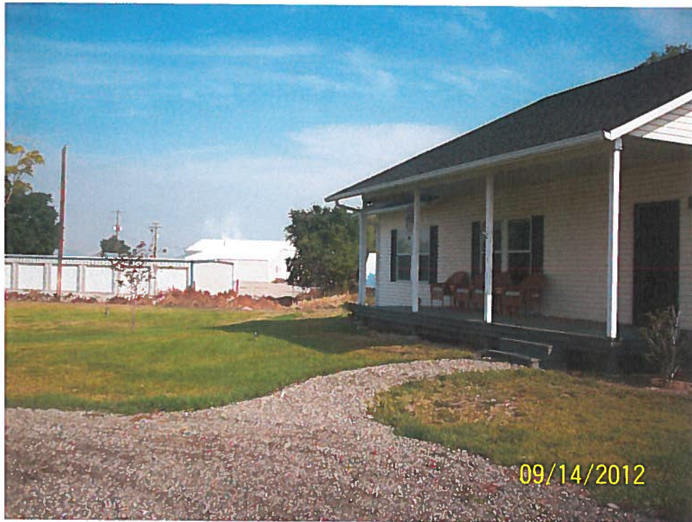
View of the front yard that show sprinkler head. (Facing North)
